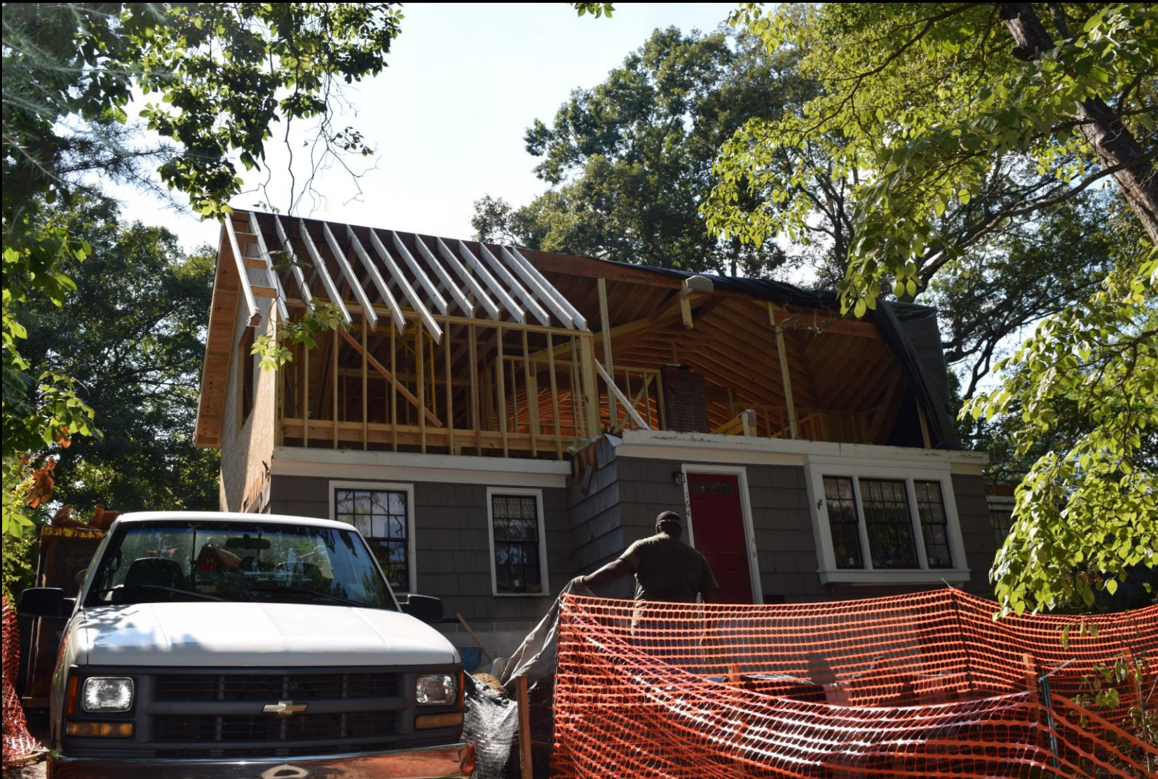
Framing has begun on the front half of the new second floor
