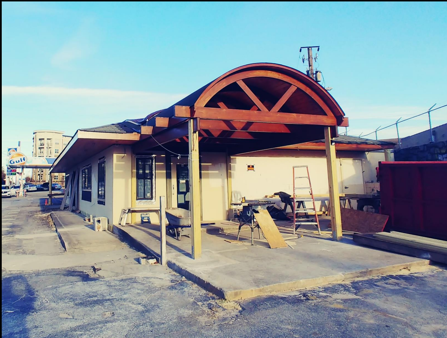
Arched Beam Trusses in place, Tongue & Groove decking installed, supporting posts installed
