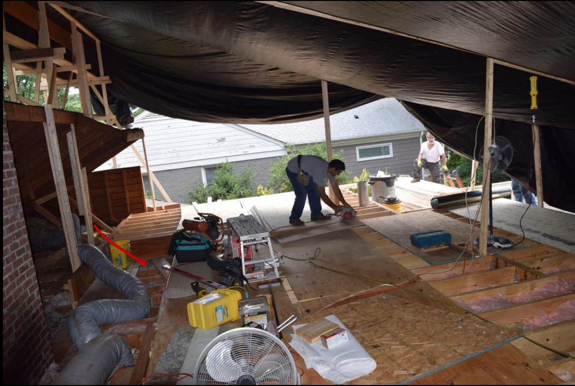
Note section of floor that has not had new joists installed and through which the flexible duct is routed. This is the location of the future stairs and stairwell.
