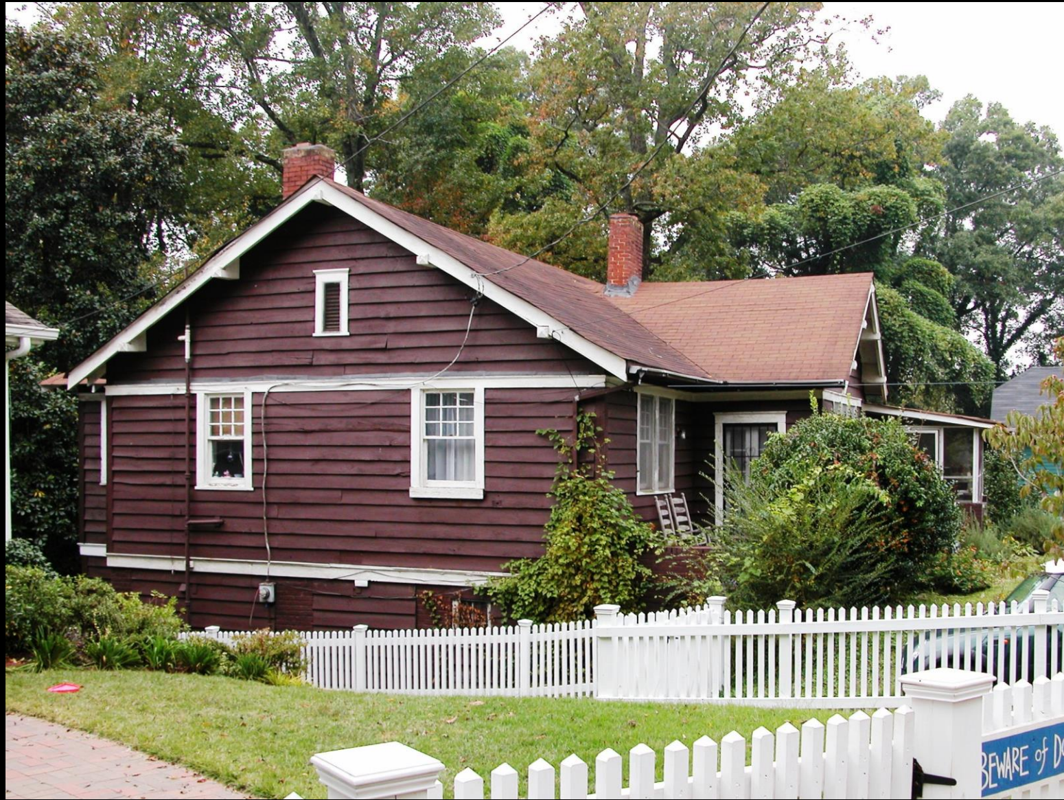
Photo of the east wall of the house before reconstruction. Note the condition of the original plank siding. There were many cracks and gaps between planks that allowed for extremely wasteful energy consumption.
