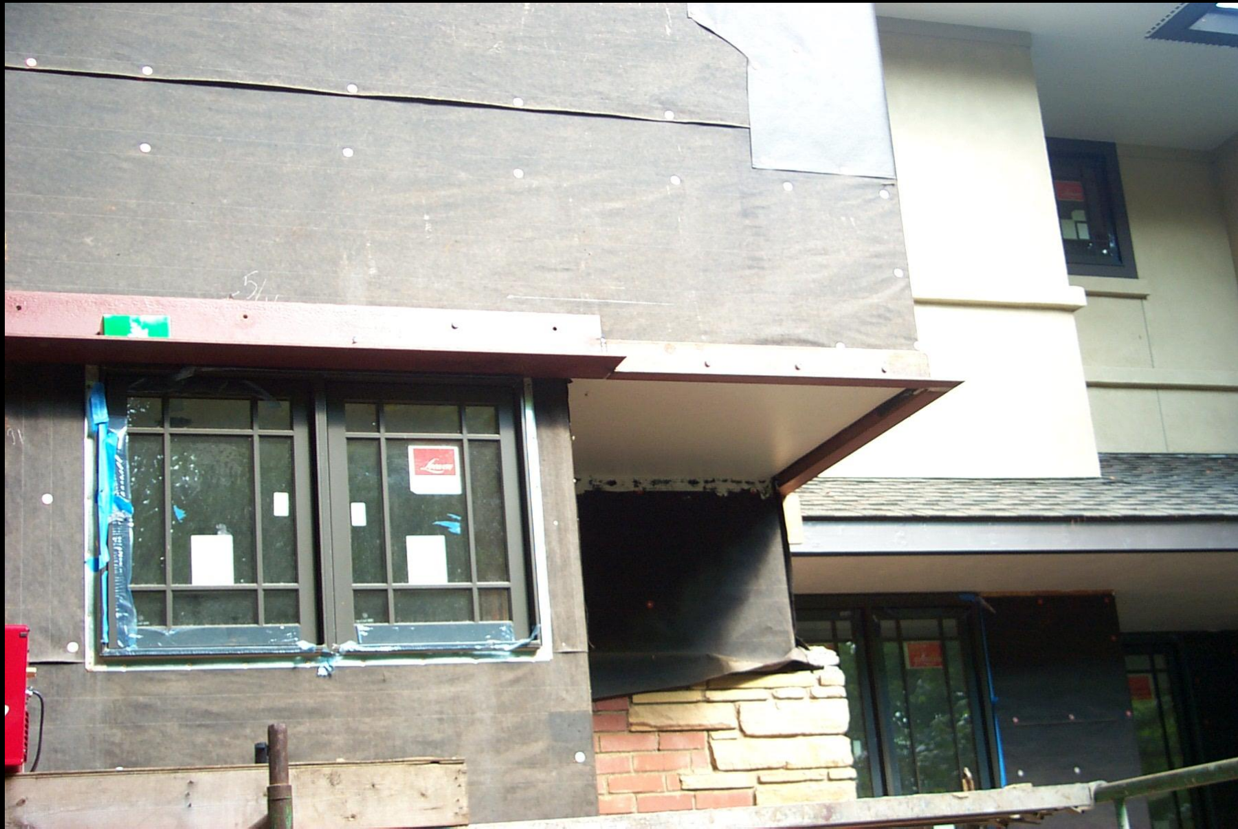
Steel channel employed to carry the second floor masonry
