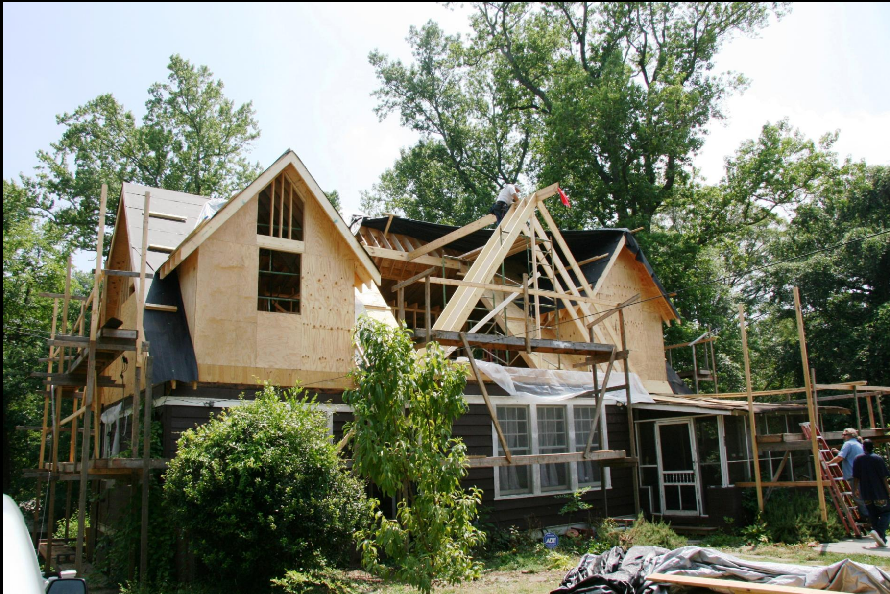
The three dormers under construction. They are the key to this design, which attempts to provide expanded functionality while remaining true to the cottage like style of the original bungalow.
