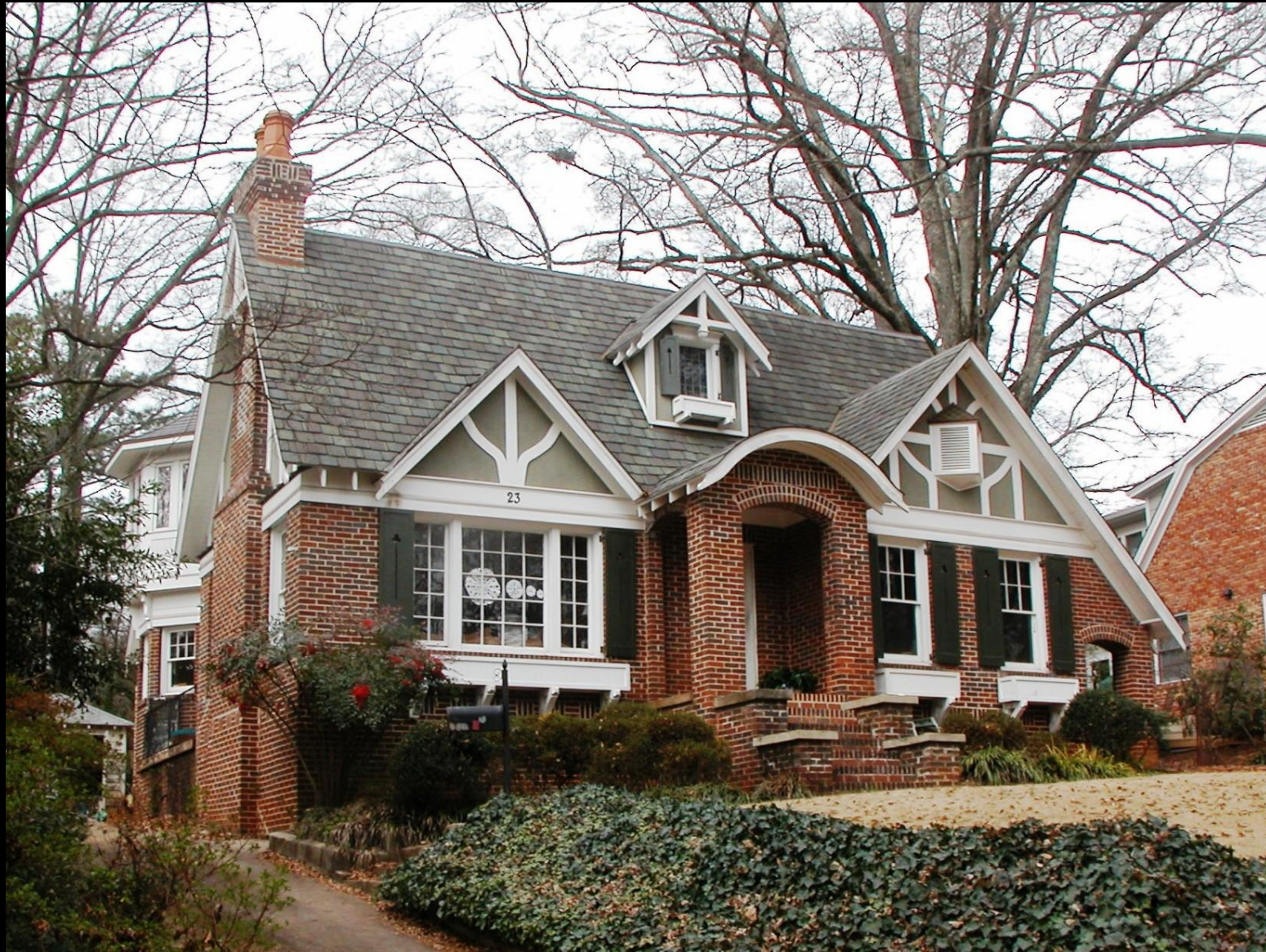
Raising the roof necessitated extending the chimney, all of which is new above the roof line. Note octagonal Master Bath with leaded glass windows at the rear
