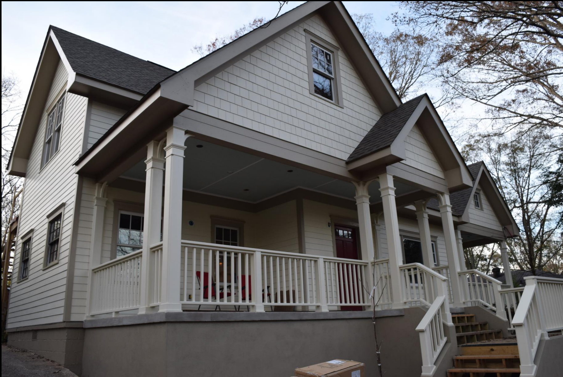
Exterior is almost complete, balustrade is in place, front stairs remain to be finished with permanent treads and risers
