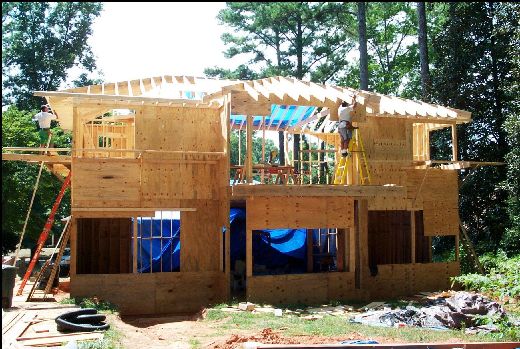
#78 Dartmouth Avenue: Wall and roof framing in place
