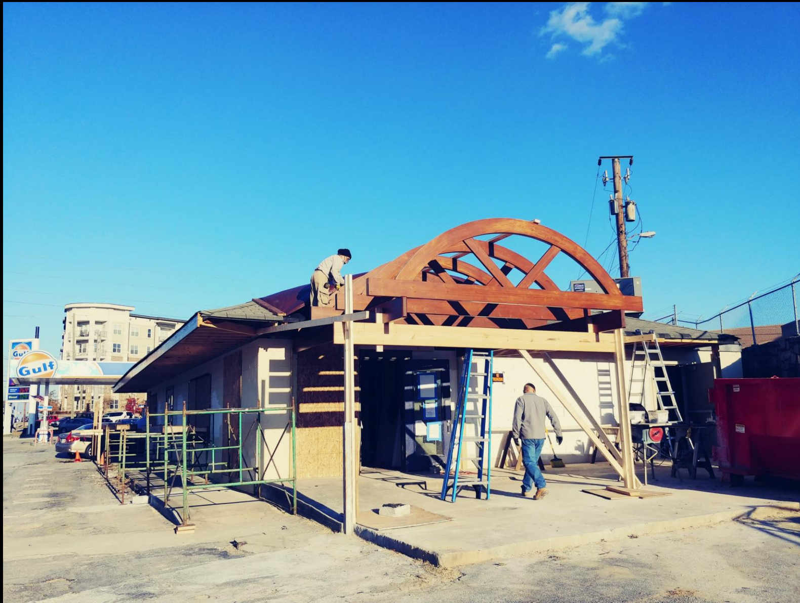
Installation of the Arched Beam Trusses
