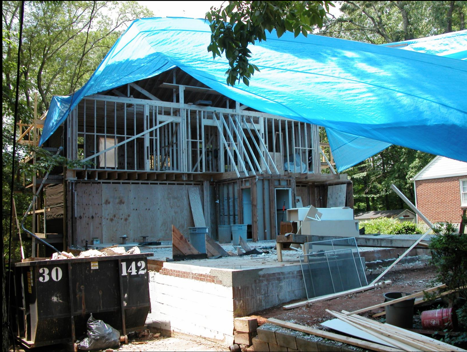
831 Stratford Rd under construction. View from the rear. Note existing foundation. Next view shows completion of framing for first and second stories built on the existing foundation.
