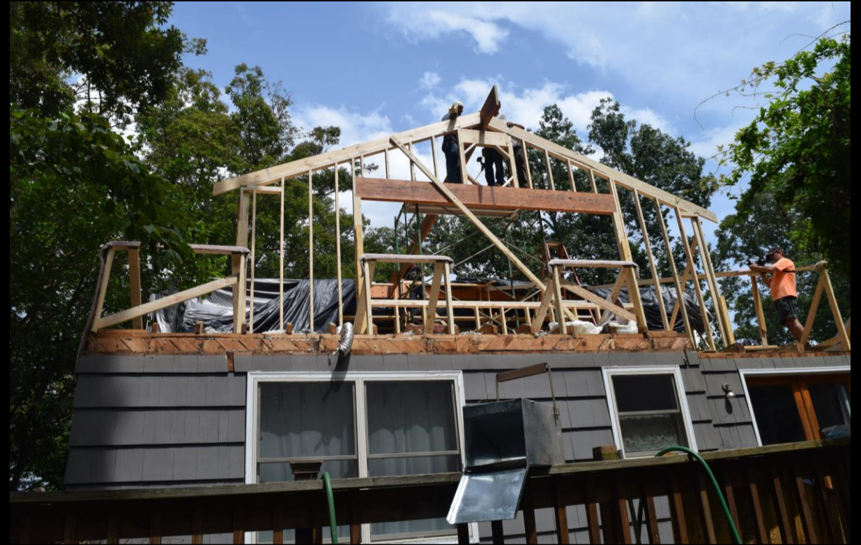
Back wall has been erected, ridge beam is being raised into place
