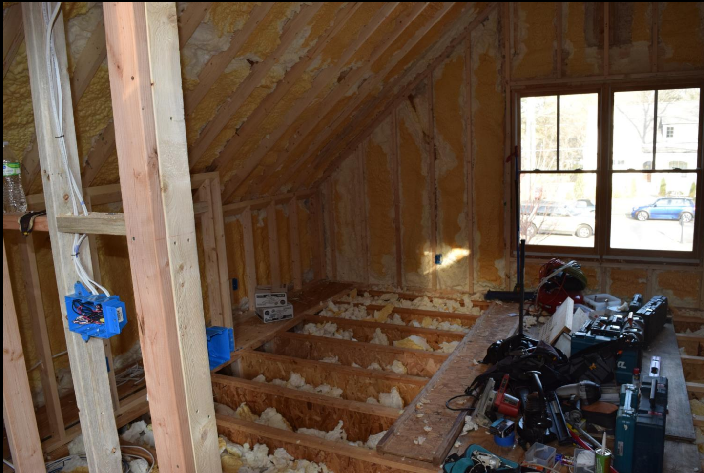
Left: View towards the front. All bracing has been removed and new knee walls have been constructed. Insulation has been placed between the floor joists since the area is now going to be air conditioned. Right: The stairway leading from the upper to the lower deck has been constructed. Caps have not yet been installed on the balustrade.
