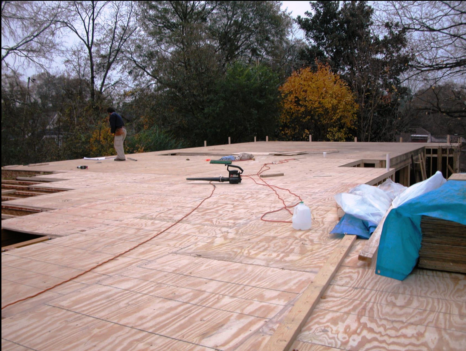
Subfloor decking being installed on the second floor
