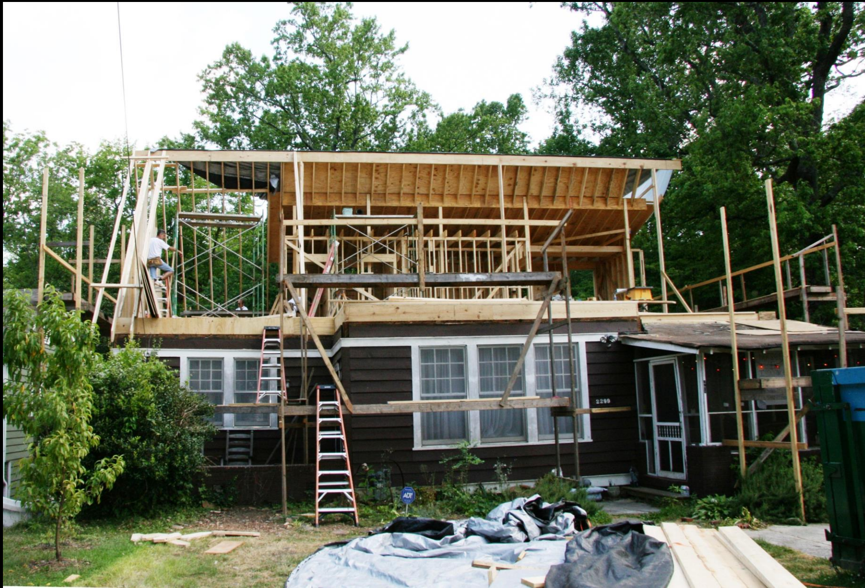
Second story roof going up. Not all projects are suitable for Owner occupancy during construction, but some do, as in this case, which involved only minimal work on the existing main floor.
