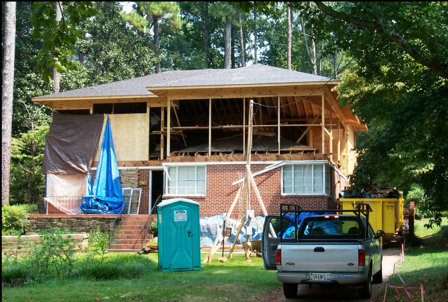
#78 Dartmouth Ave. reconstruction in progress. Note how the new roof is constructed over the existing roof. After removal of original roof second story walls will be constructed. A new second story floor system will be constructed independent of the existing ceiling and will be leveled to within 1/16 th of an inch over the whole house.
