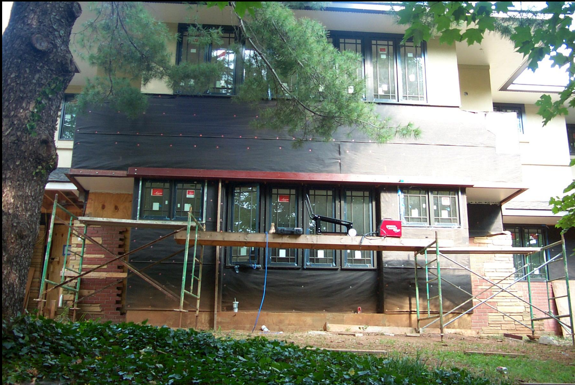
Cantilevered steel channel employed to carry the second floor masonry
