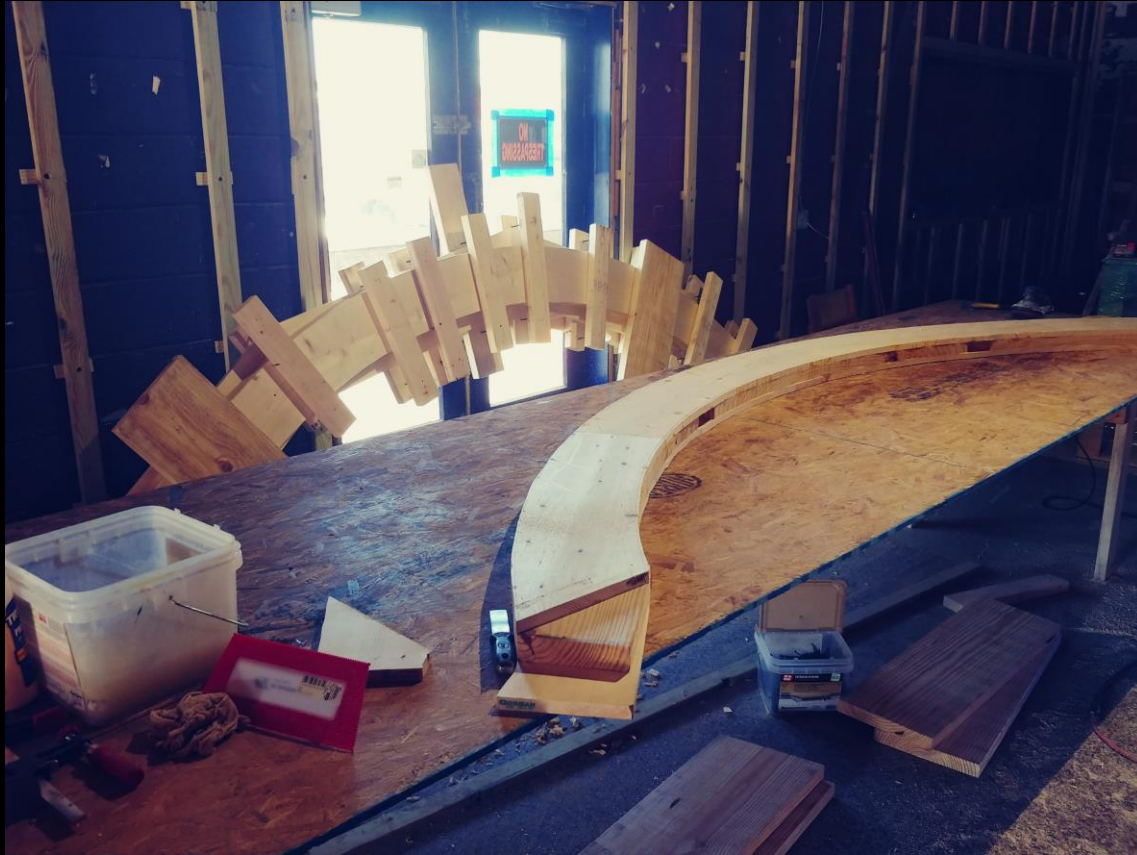
Construction of arched beams for the barrel vault entrance
