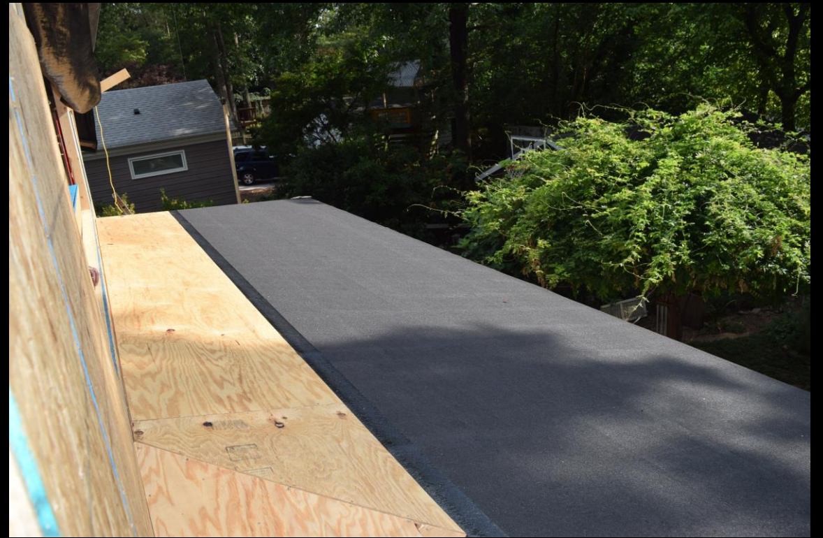
Role roofing being installed
