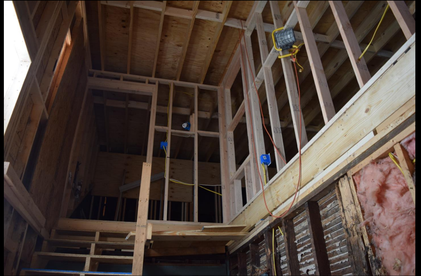
Left: Stairs and stair well roughed-in. Above: The stairwell will be the only finished space in this project. As with all second story additions, the new floor is independently leveled with respect to the existing walls and ceilings.
