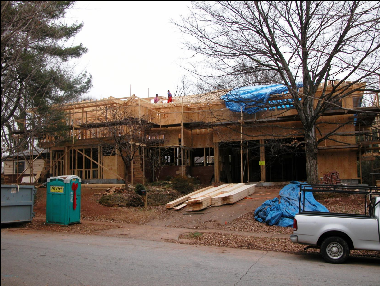
Second floor walls have been constructed and roof is being framed
