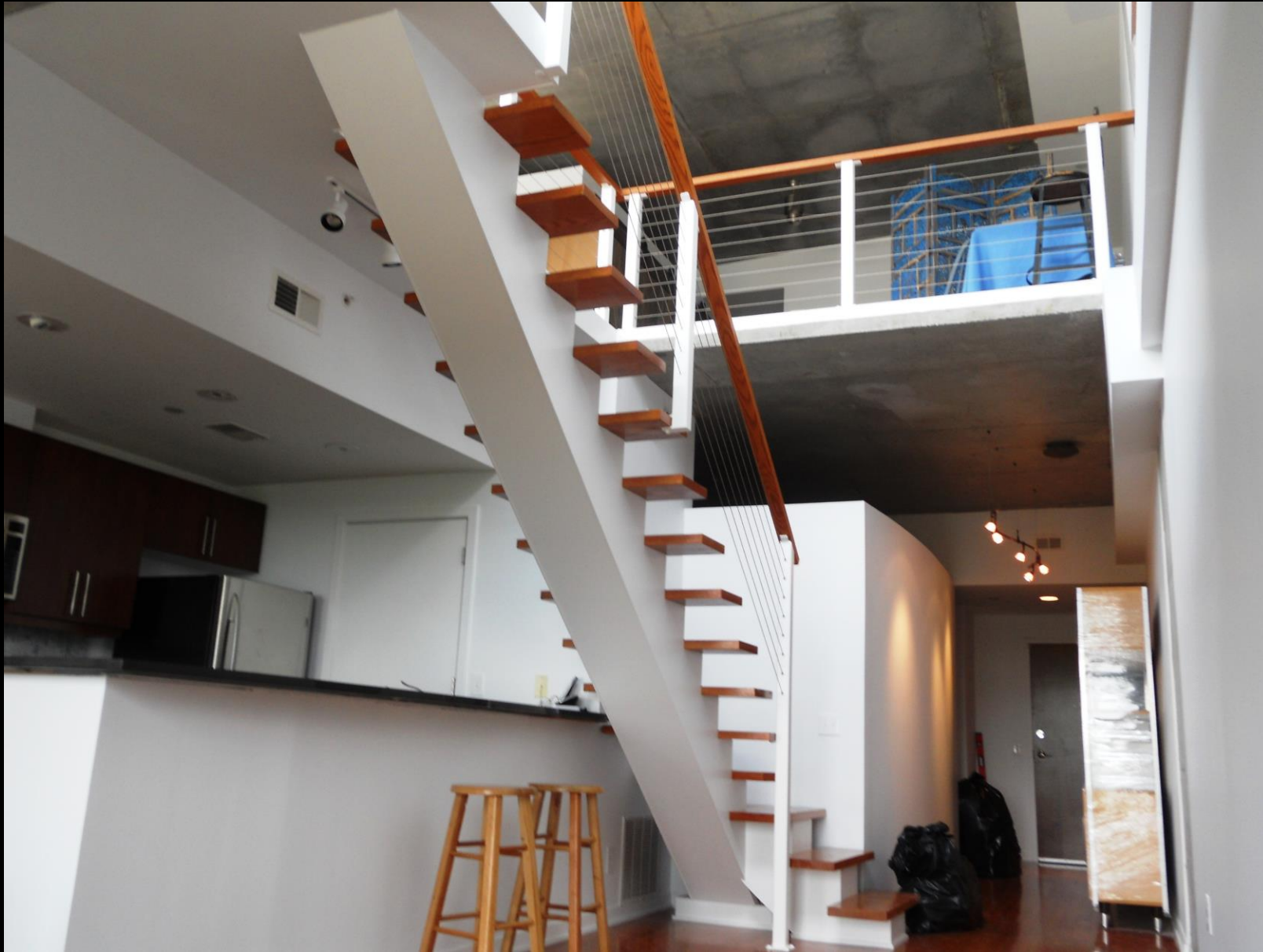
Loft project with open plan stairs with cable railing
