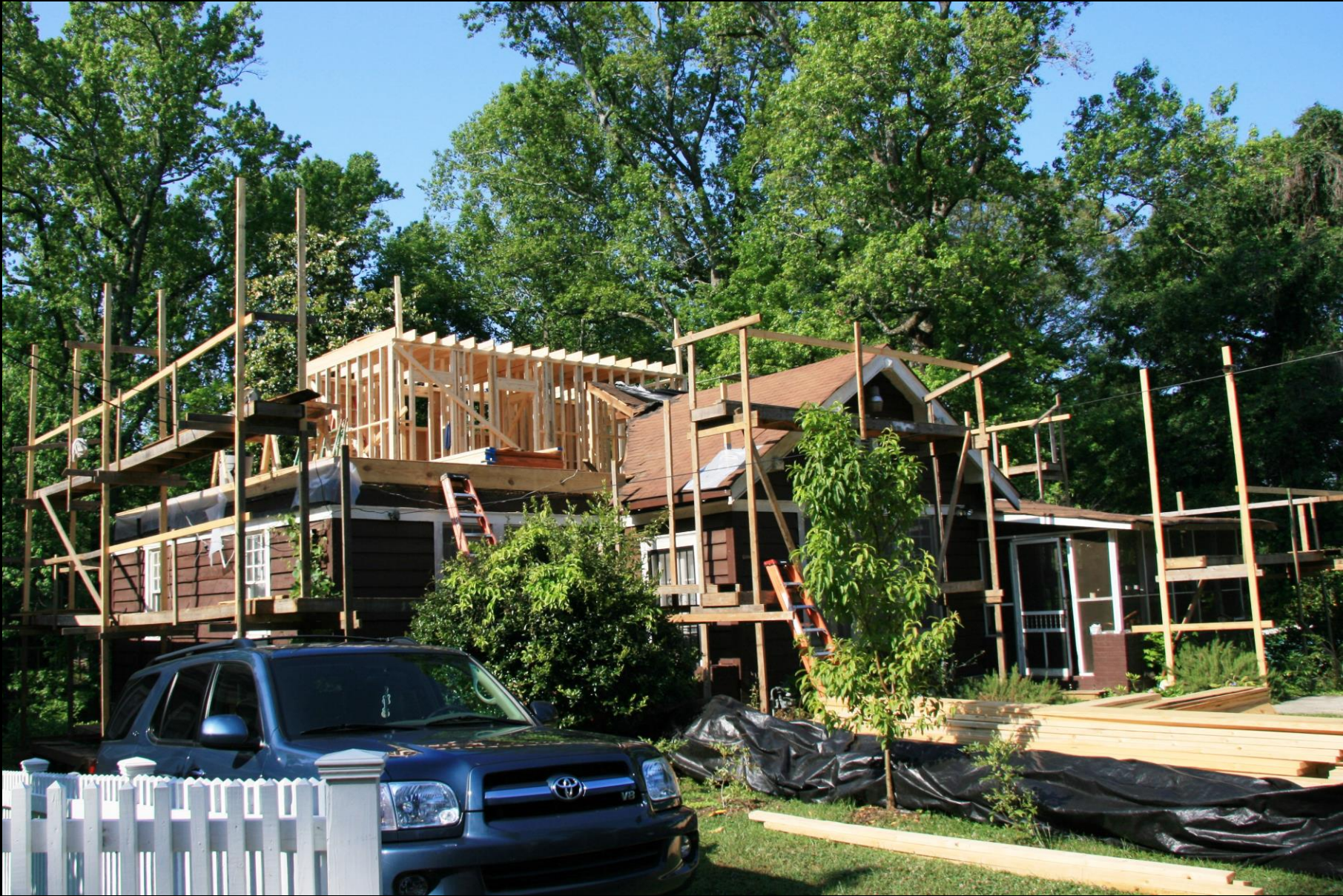
2299 Cottage Grove under construction. The first walls of the second story are going up. The Owners lived in the house below throughout the entire process, which, for the most part is going on entirely outside of their living space. Only at the end of the job do we break through in order to build a staircase to connect the two floors.
