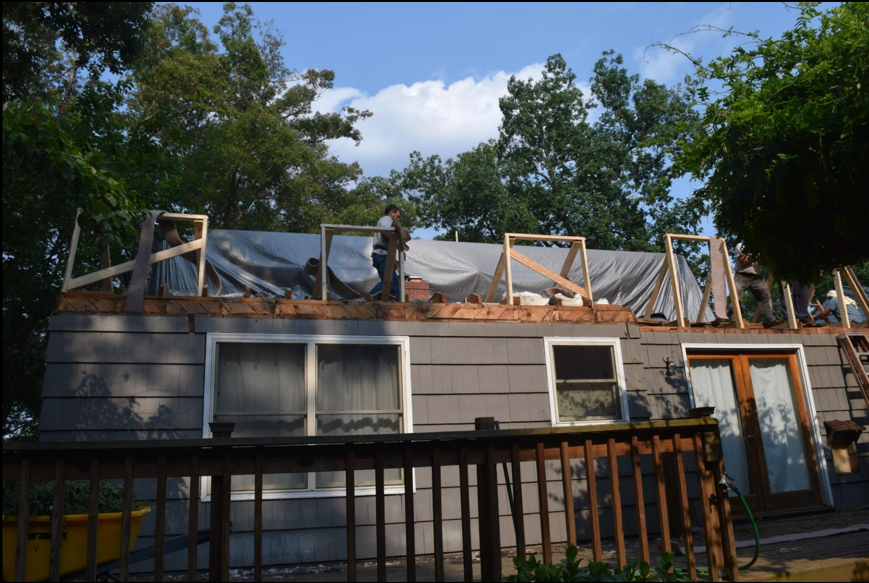
The temporary supports for the tent are in place. Once the roof is dried-in the tent will be removed.
