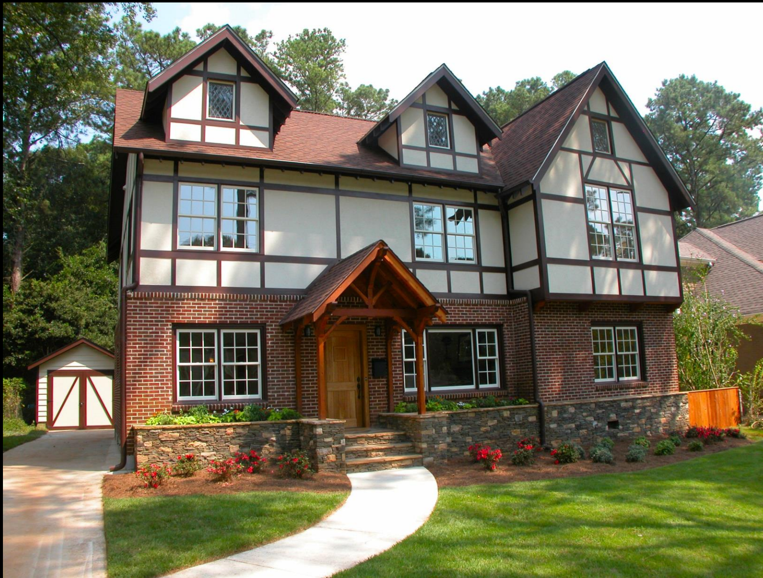
The complete project. Note the leaded glass windows in the gables. The stucco system is a 3-coat hybrid with traditional base coat troweled onto steel lath, a second scratch coat and a top coat of pigmented acrylic. This creates a long lasting, low maintenance surface.
