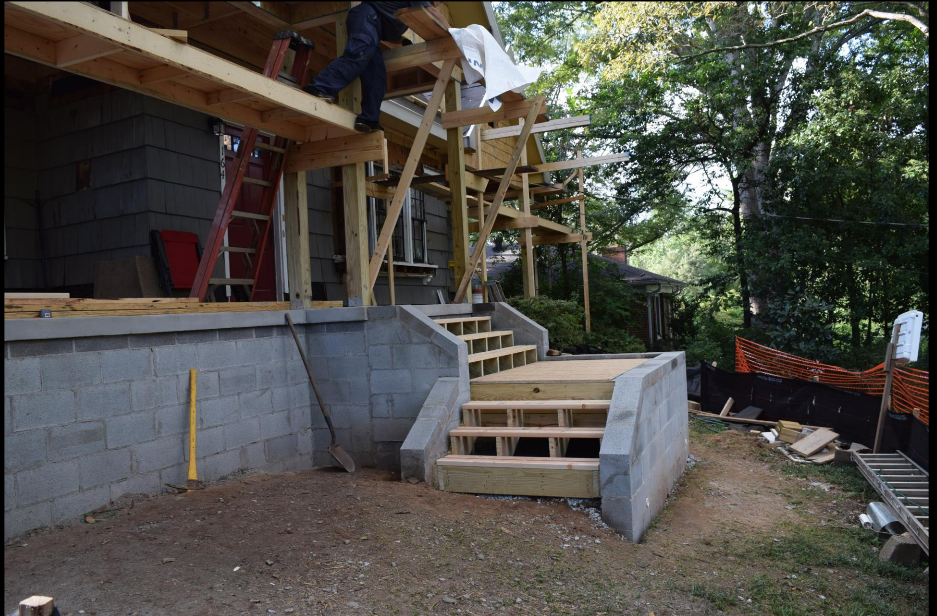
Front stairs: Masonry and framing carpentry complete
