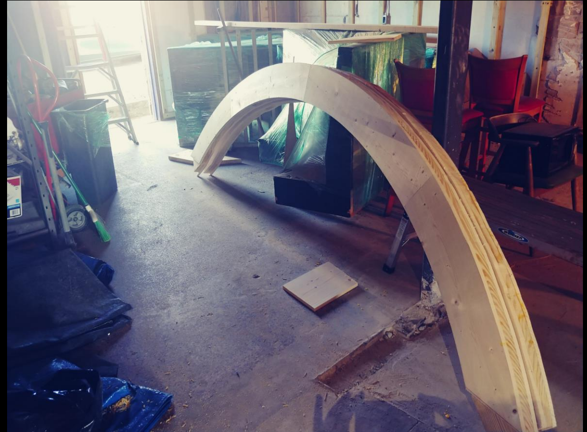
Construction of arched beams for the barrel vault entrance
