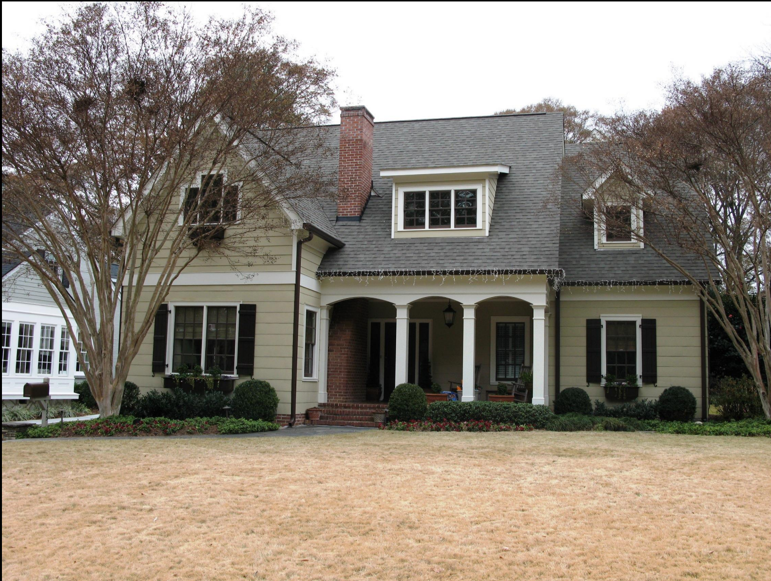
Lamont Drive after reconstruction. Note increased height and pitch of the roof and the addition of two dormers, one with a shed roof and the other with a gable. Note also on the front facing wing how the roof has been raised to accommodate a third upstairs bedroom. Note also the improved portico with new columns and arched lintels.
