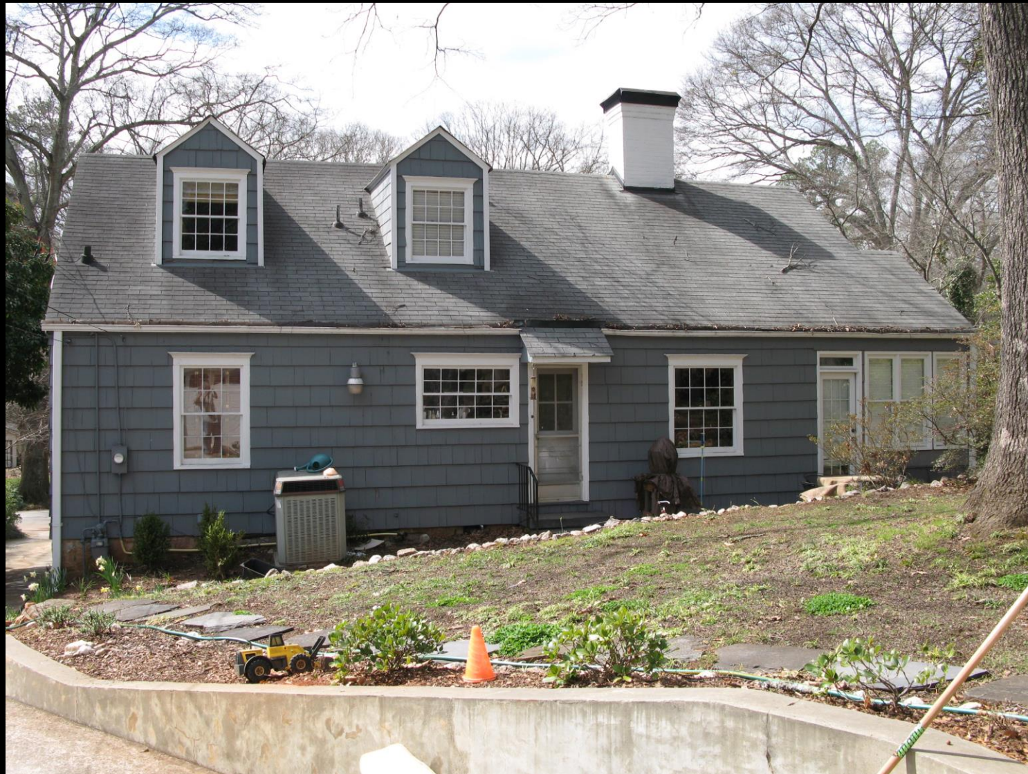
#28 Dartmouth Avenue, Avondale Estates, Georgia. Rear, east facing wall prior to redesign and reconstruction. The idea was to punch out the kitchen by 12 feet. The wide window with 5 horizontal panes looks into the kitchen which is going to be expanded outward toward the rear. Wall removal will encompass both the window and the rear door. The window to the right of the door will open into the new screen porch.
