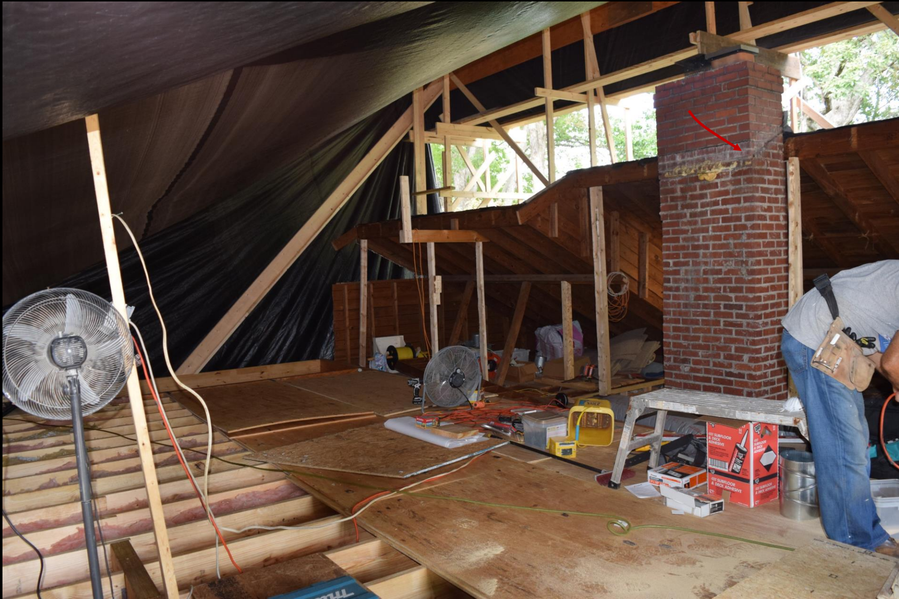
Tent is in place, back half of the roof has been removed, new floor joists are in place. Note front half of the original roof is still in place. Note that the old roof line is still visible on the chimney.
