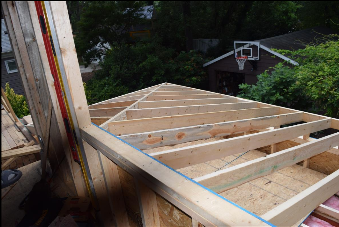
Framing the roof for the new single story first floor
