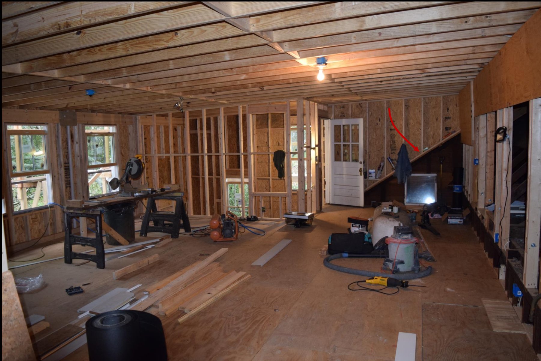
The new space is taking shape. Owners elected to not finish out the space as its primary purpose was storage. However, the room could be finished at a later date by current or future Owners. Note door to the stairwell and the original roof line which is visible in the far wall as indicated by red arrow.
