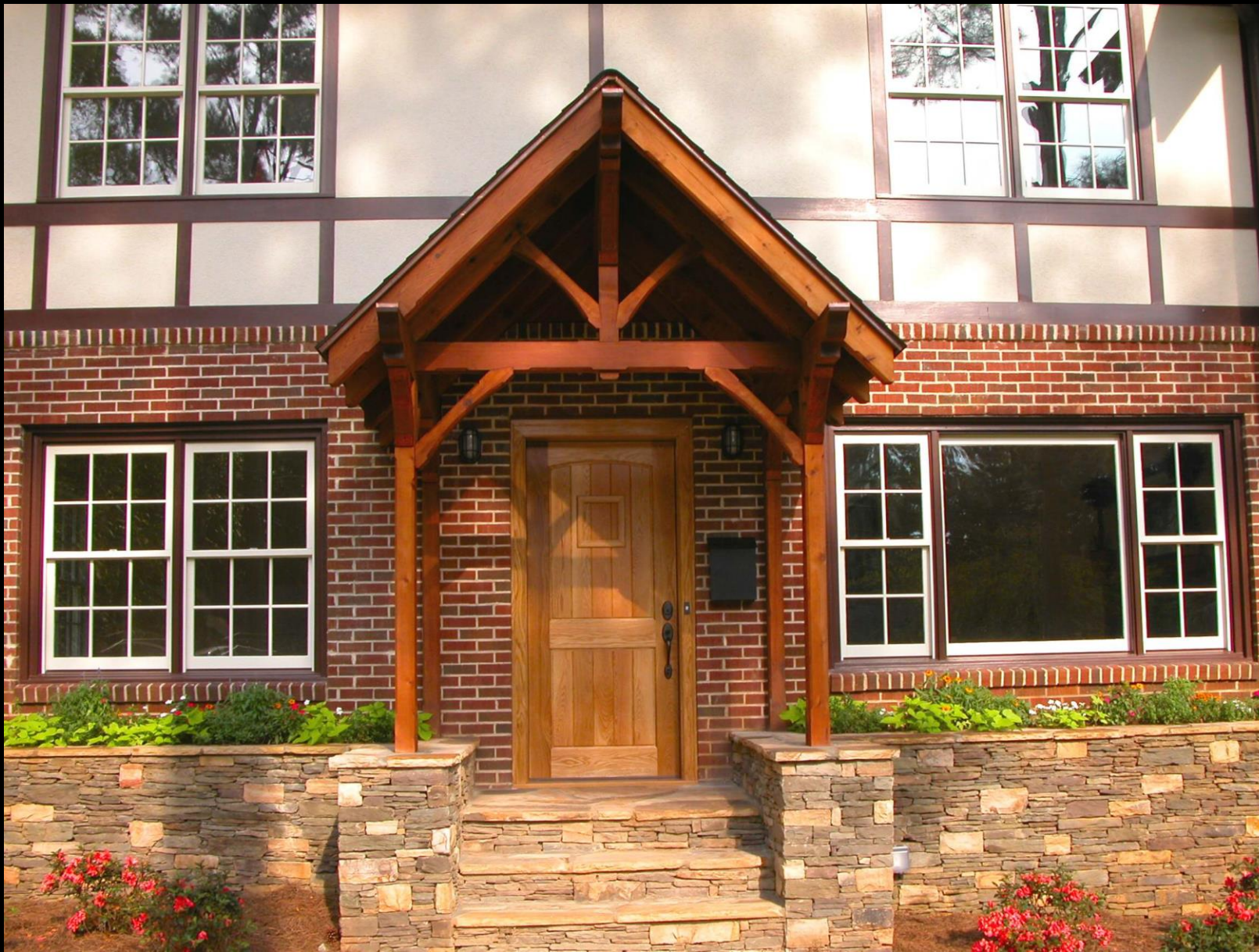
Front entryway with timber framed portico and custom-built oak door with operable 'speakeasy' window
