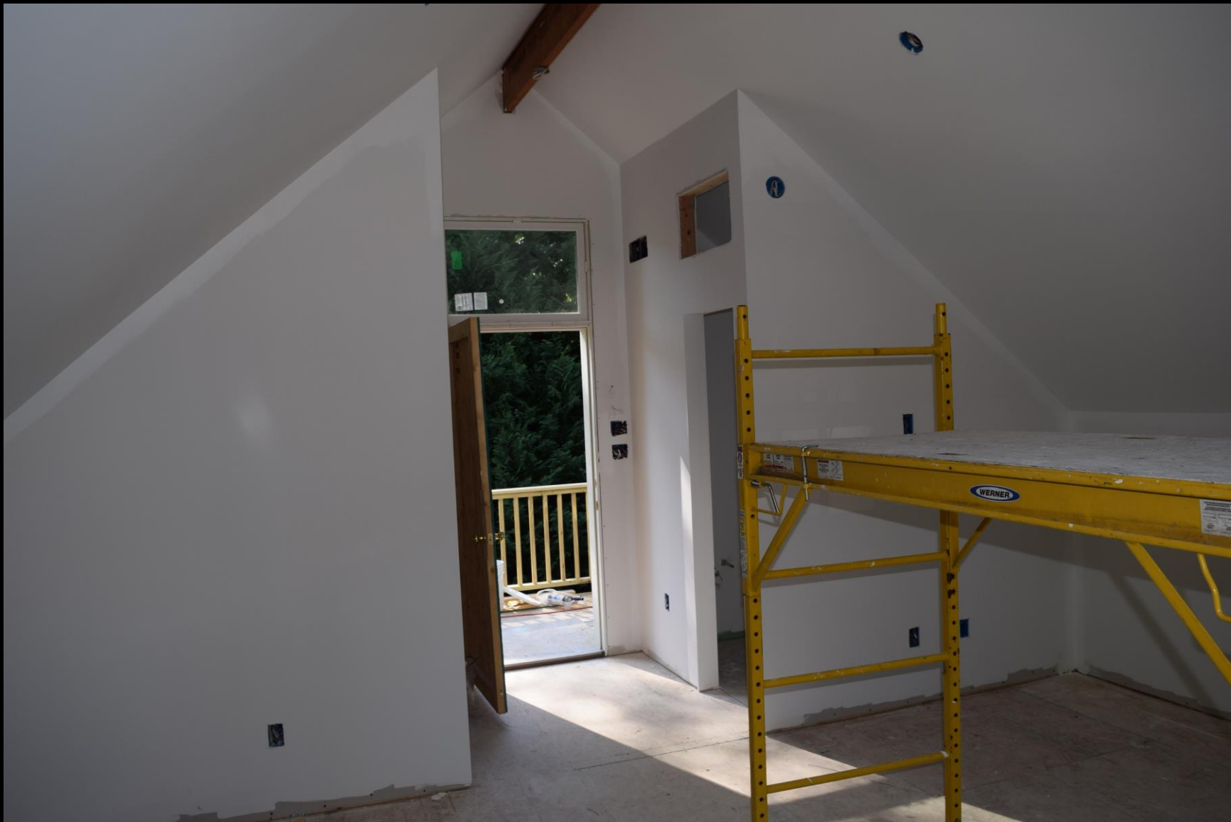
Drywall has been installed, taped and primed. Note exposed glue-lam ridge beam.
