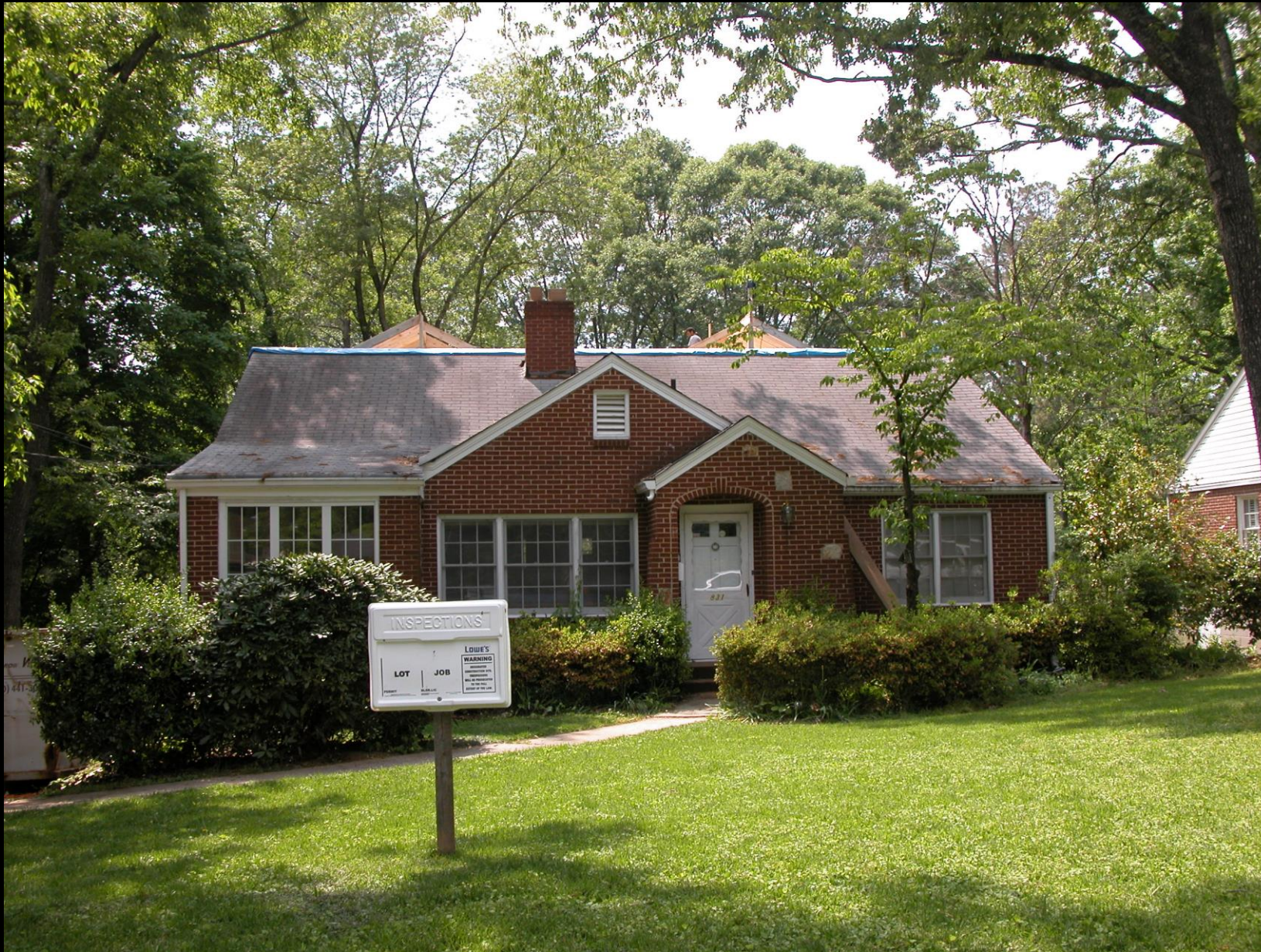
831 Stratford Road, Avondale Estates, Georgia. This house was built during the interwar years and suffered major deficiencies. The mortar of the brick was deteriorated and the framing/rough carpentry was substandard. However, the foundation was in extremely good condition and well-built. The decision was made to build a new house on the existing foundation, utilizing the same footprint in the new design.
