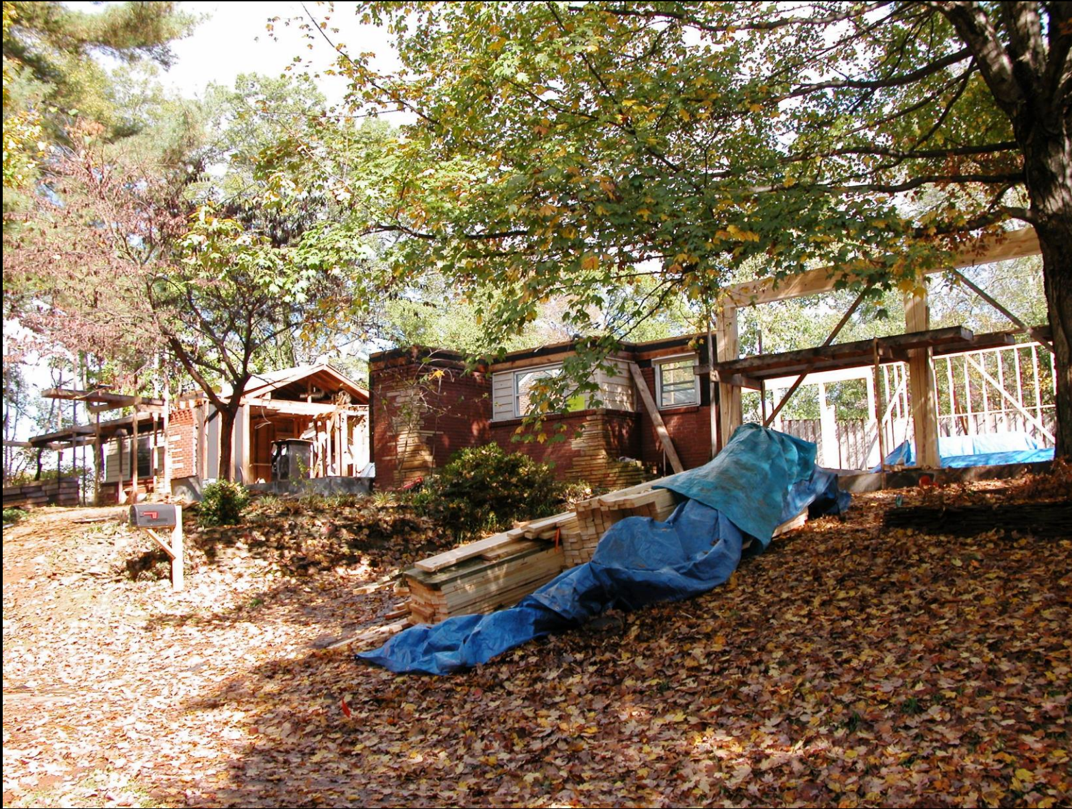
#2 Dartmouth during reconstruction. Note that only sections of the masonry façade remain. All existing walls and other structure has been removed and new walls, floors, ceilings and roof are being entirely replaced with new framing.
