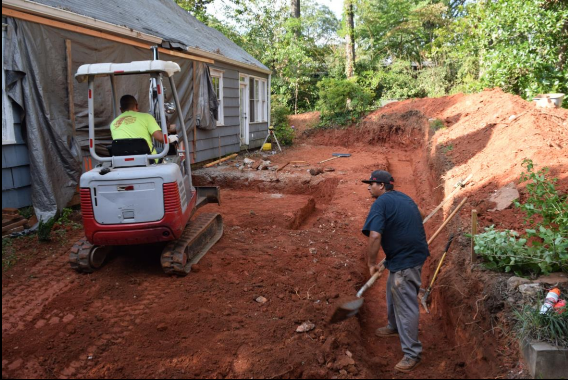
Excavation has begun. Footing trenches have been dug for the foundation of the kitchen extension and for the 62 foot long retaining wall. View looking north
