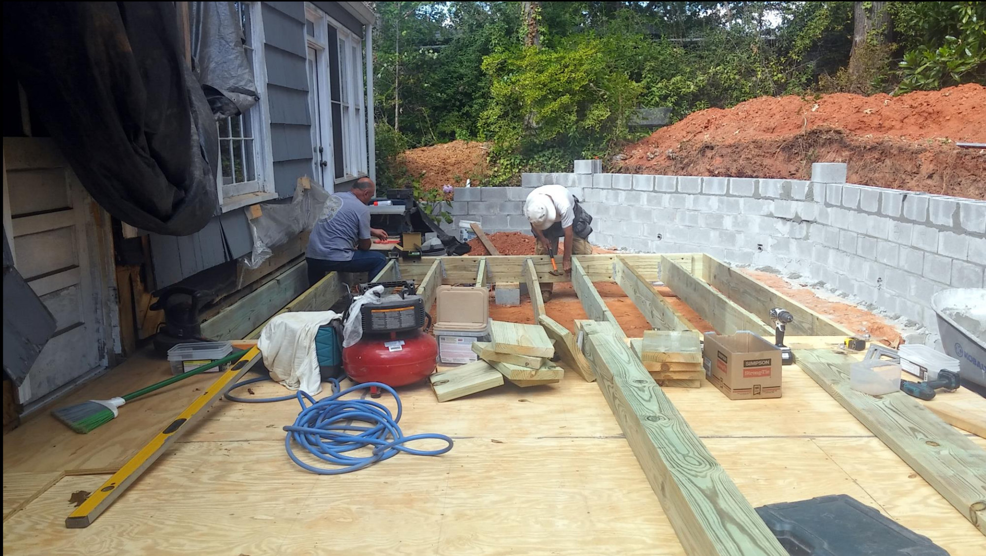
Retaining wall is nearing completion, new kitchen floor is decked and carpenters are framing the floor for the new screen porch
