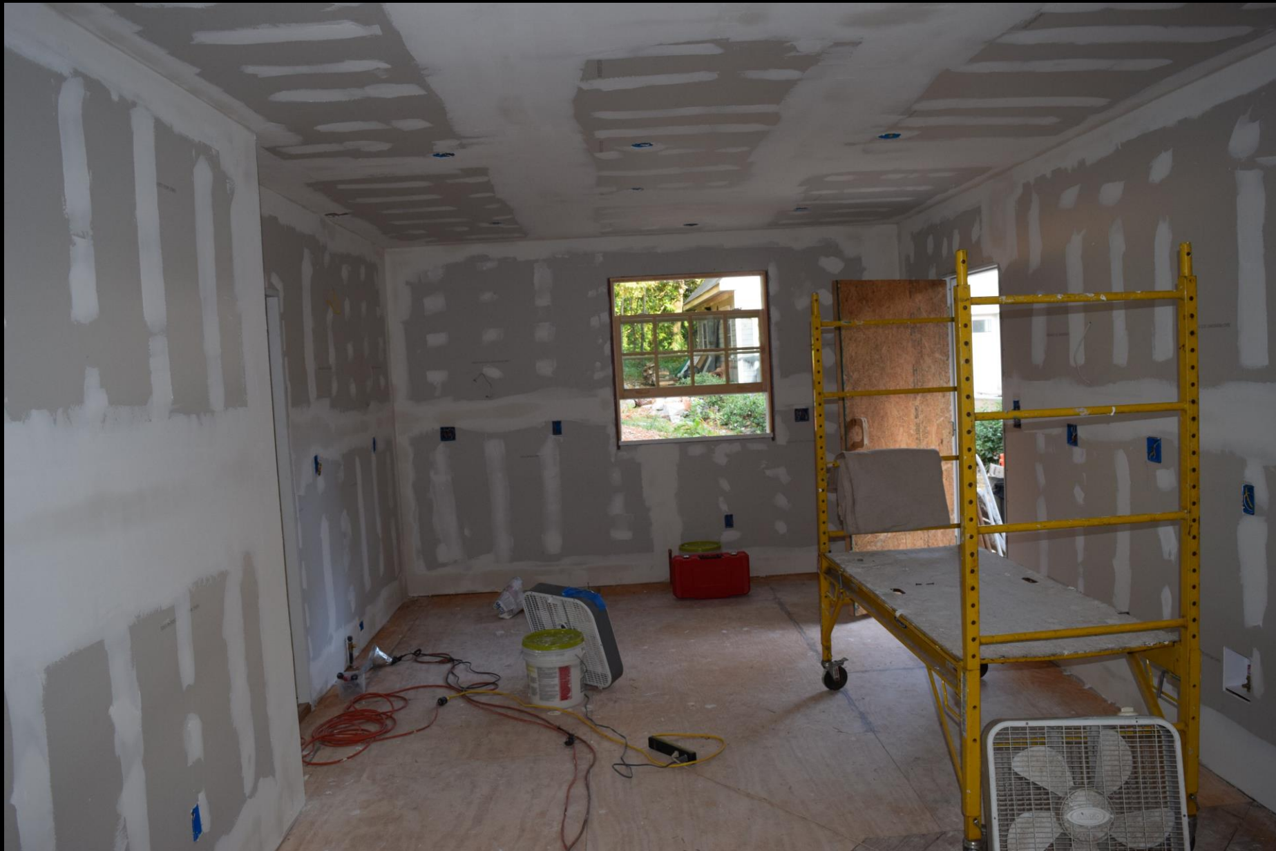
Same view as previous slide. The back wall of the original kitchen has been removed to open up into the 12 foot extension.
