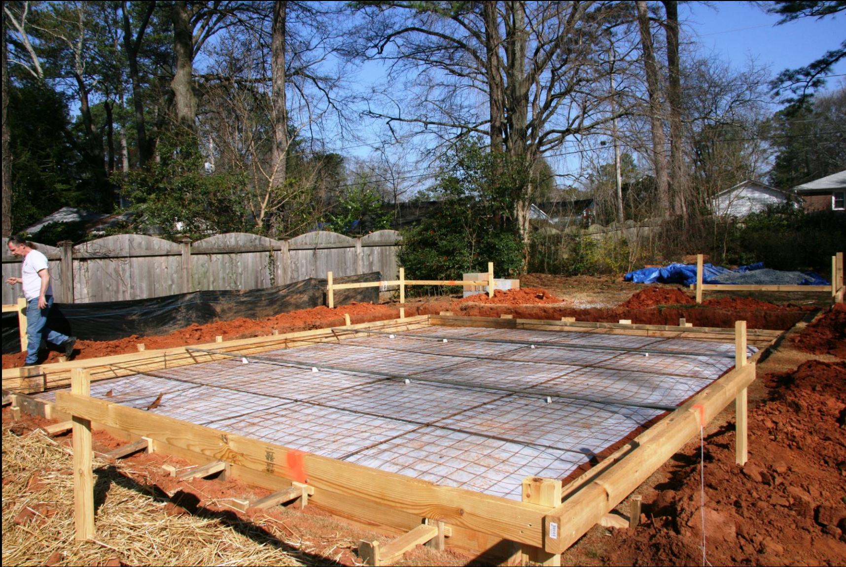
#2 Lakeview Place Garage/Office – Ready to pour the slab with integrated footings. Note presence of both welded wire mesh and #4 rebar throughout the slab.
