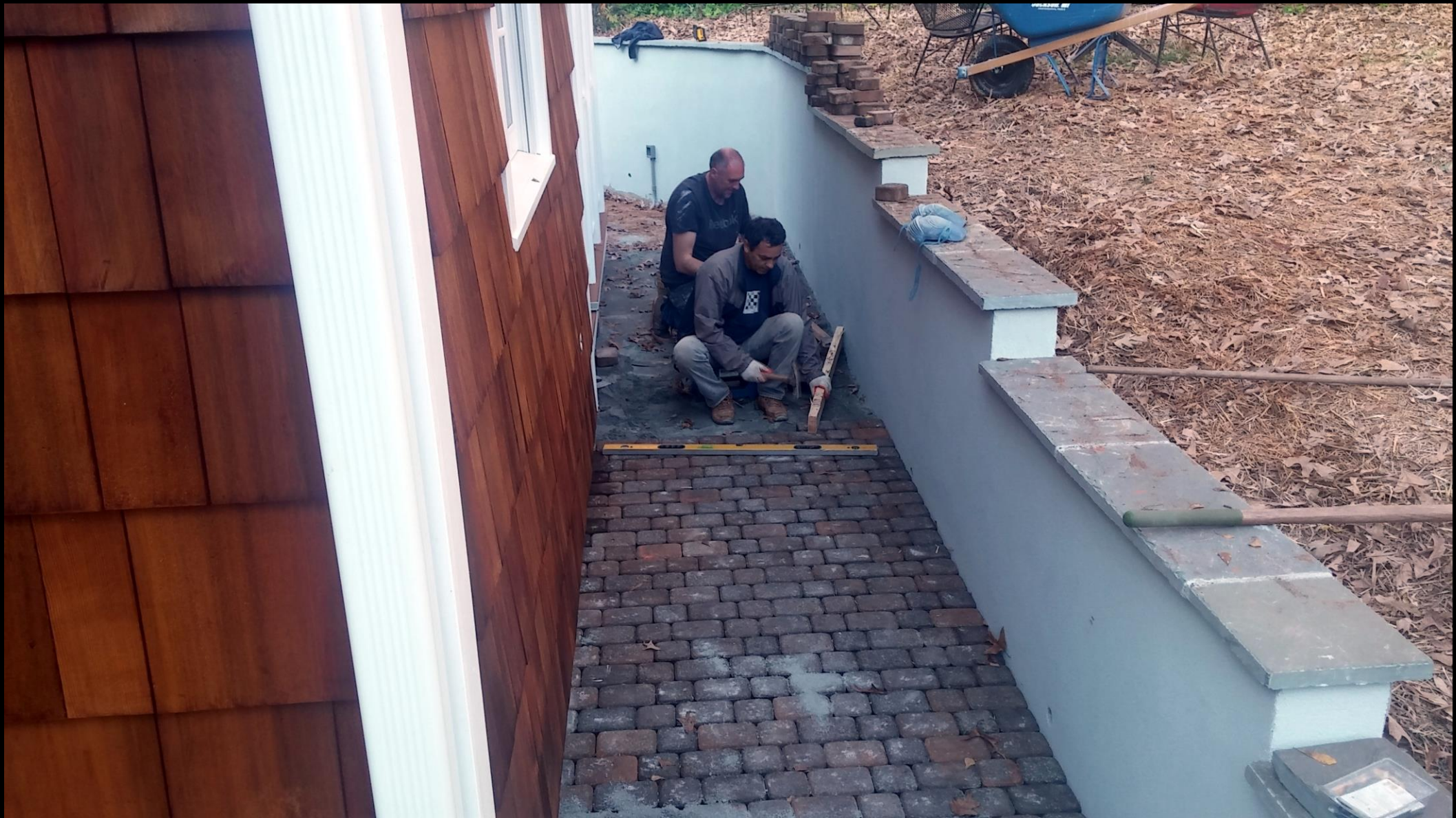
Installing the paving blocks around the perimeter of the new kitchen addition and porch. Stucco finish and capstones have been applied to the retaining wall.
