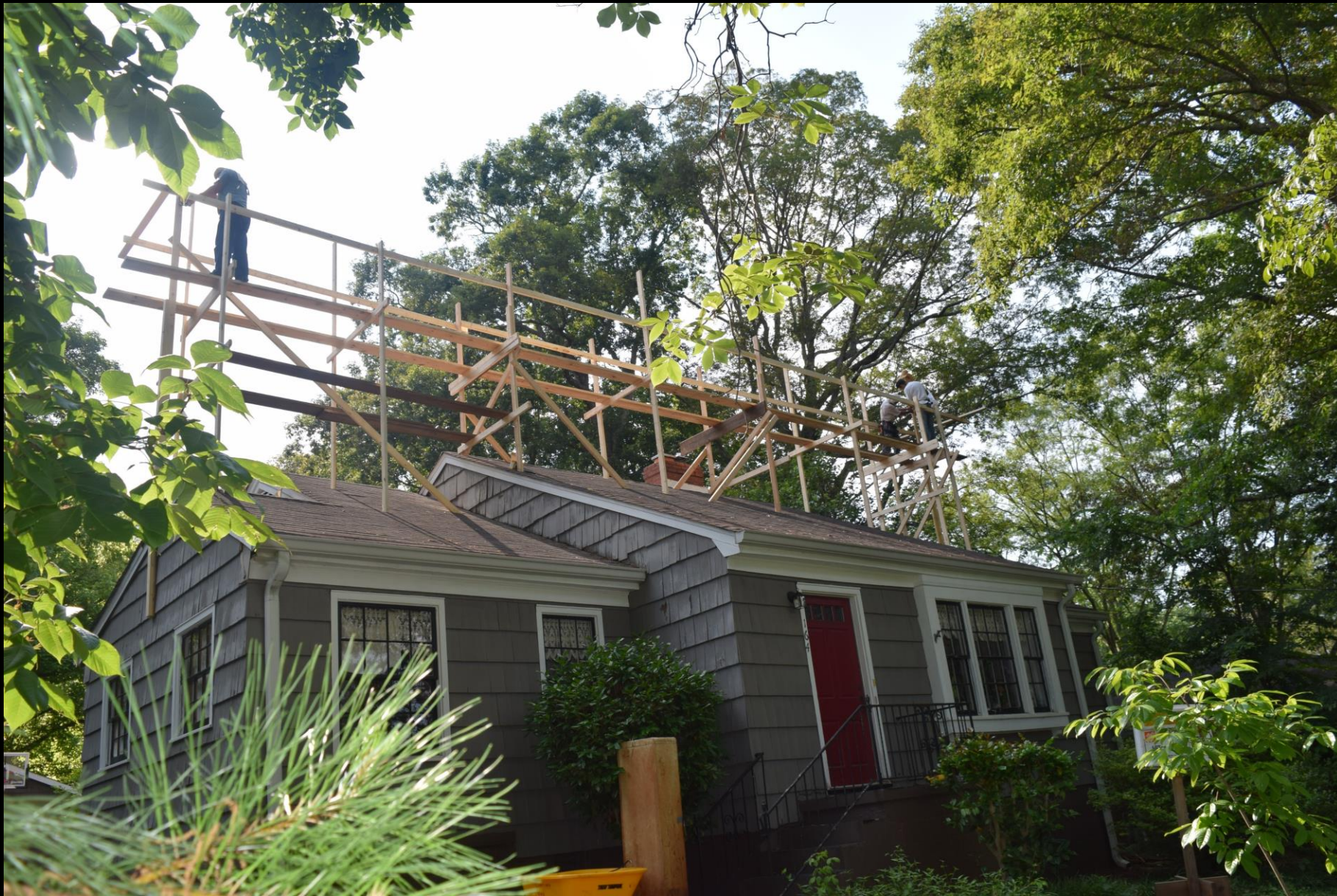
First stage of the work: Erection of scaffolding in preparation for raising the ridge beam and construction of a temporary canopy over the house.
