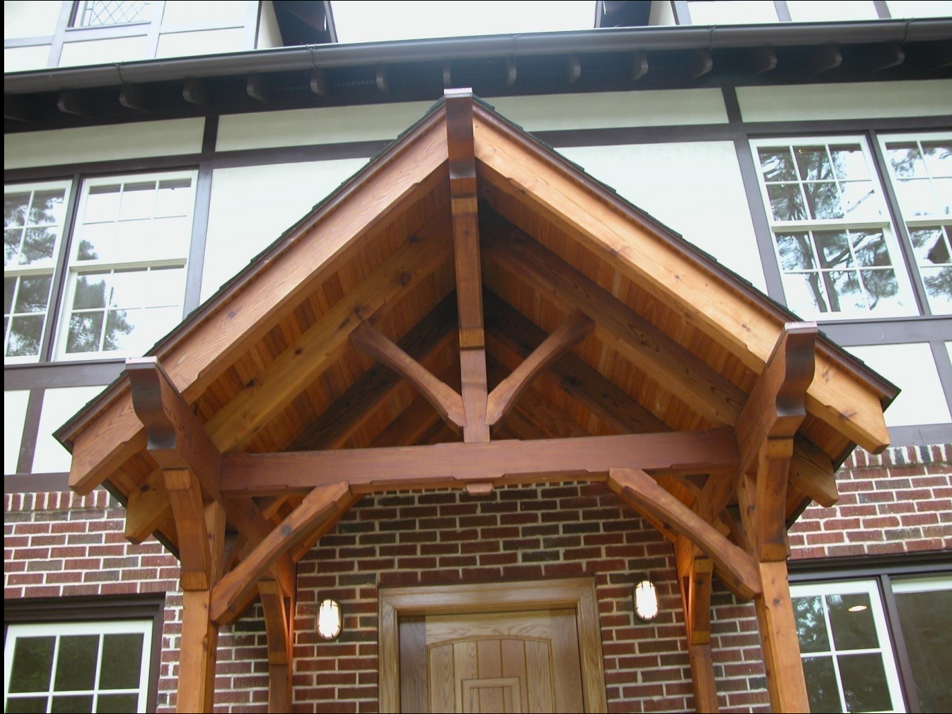
Timber framing details on the front portico
